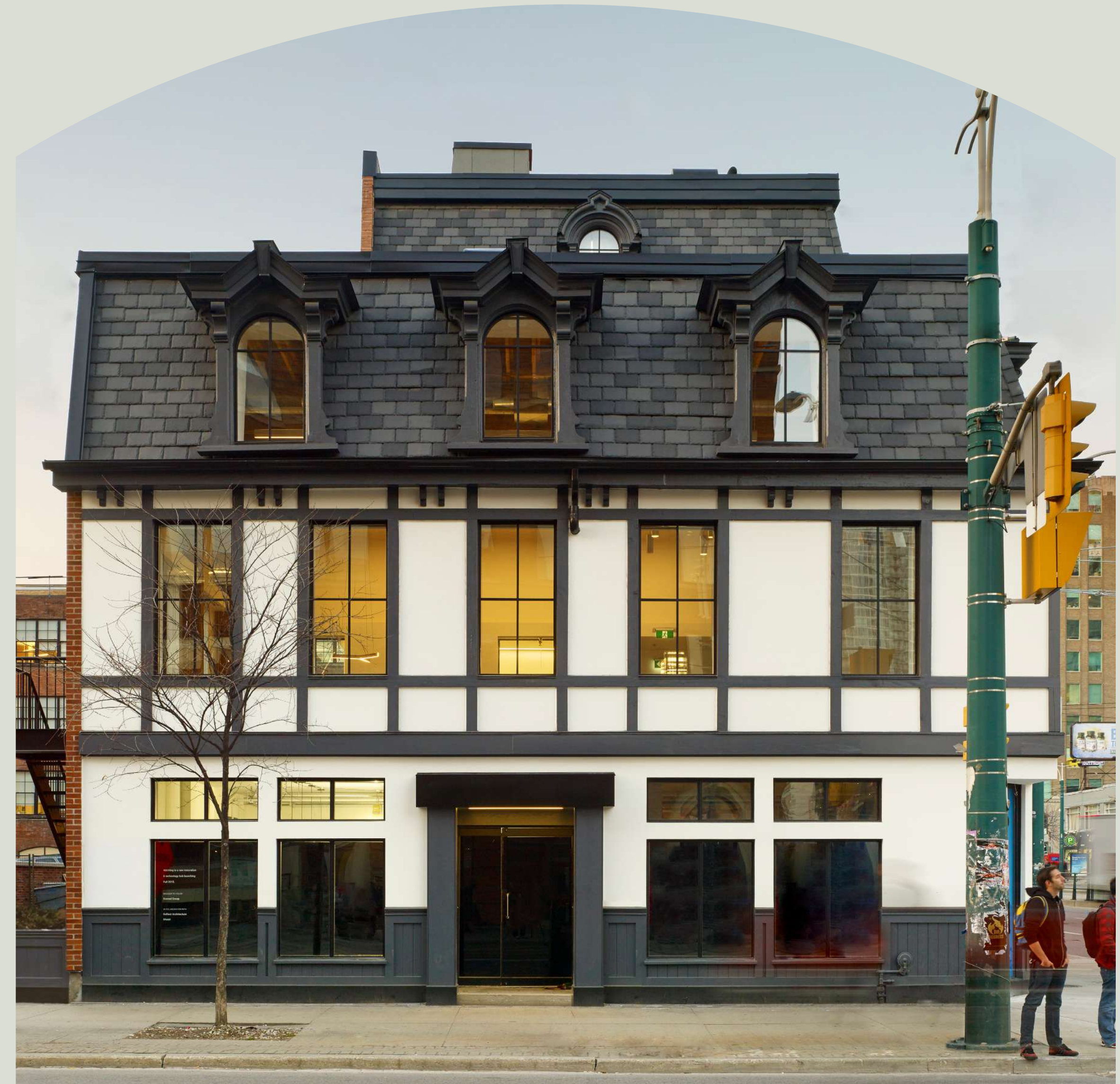
460 King Street West's southern facade
